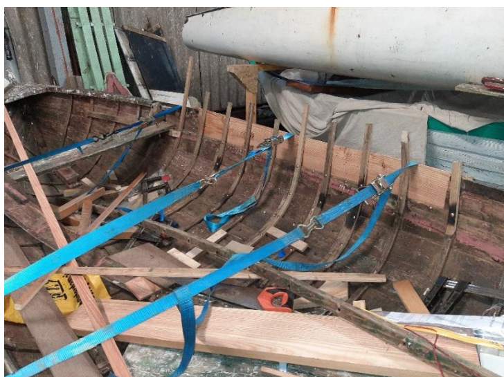
Figure 44 - Top stroke and timbers reinstated
