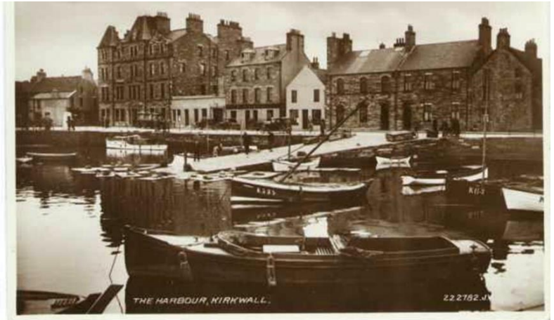
Figure 18- Nellie (foreground) in Kirkwall Basin 1920
