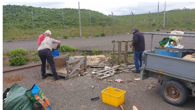
Removing inherited rubbish from the rear compound
